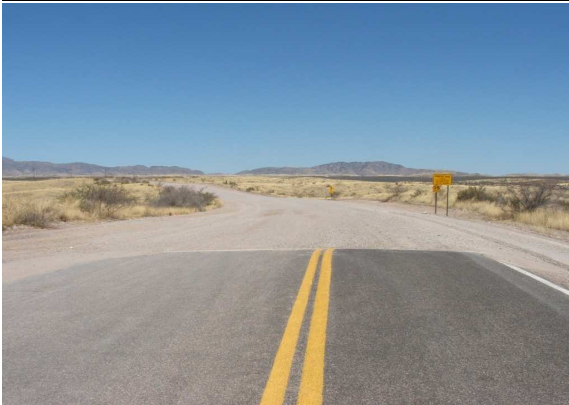
Gleeson Road (west termini) looking East.
