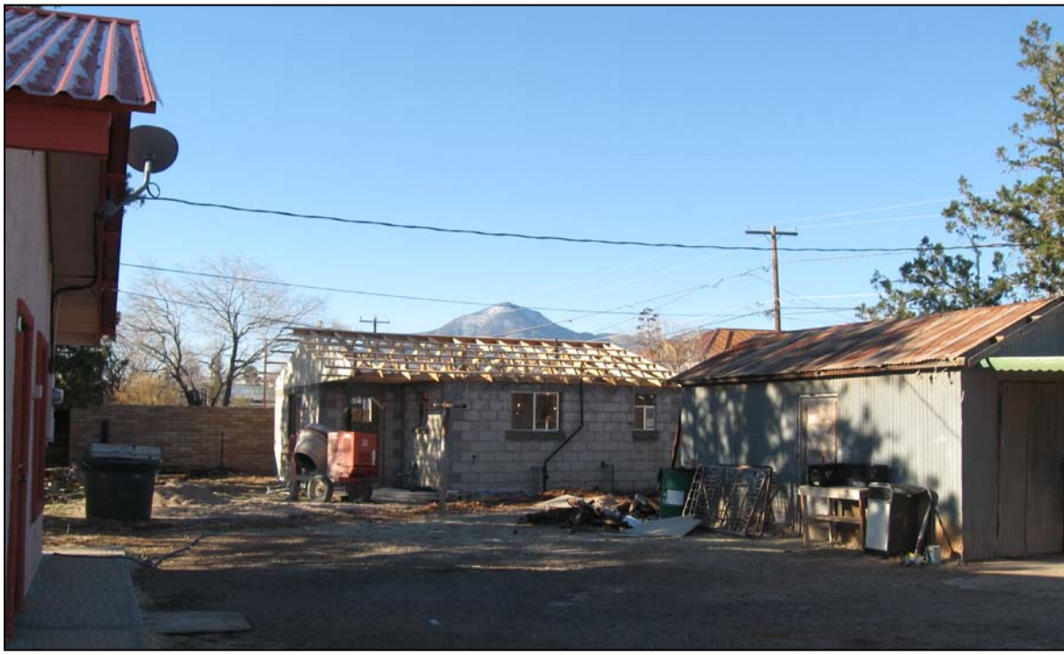
The proposed second dwelling and storage building. Existing residence at left.
