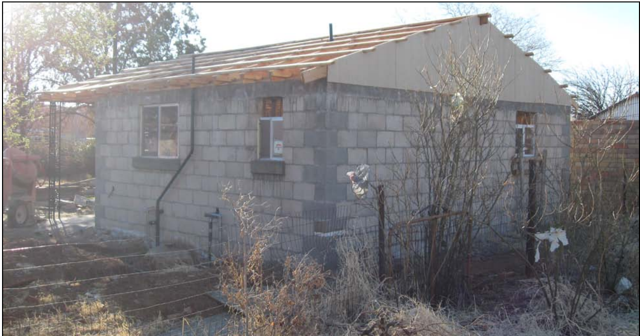
Southeast view of the partially-constructed second dwelling.
