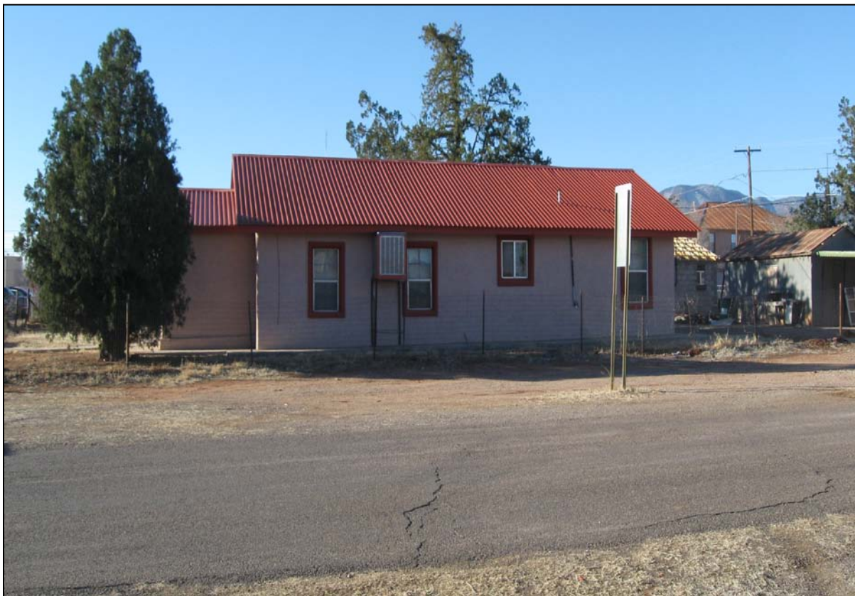
South view of the Yesca residence, seen from Valenzuela Street.
