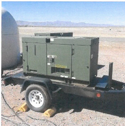
15 KW Generator 7 ft long x 5 ft tall x 4 ft wide
