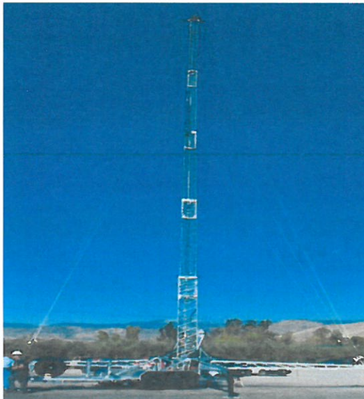
Tower 62 ft tall x 20 ft base
