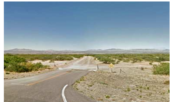
Existing Post Ranch Rd. Intersection with SR92.
