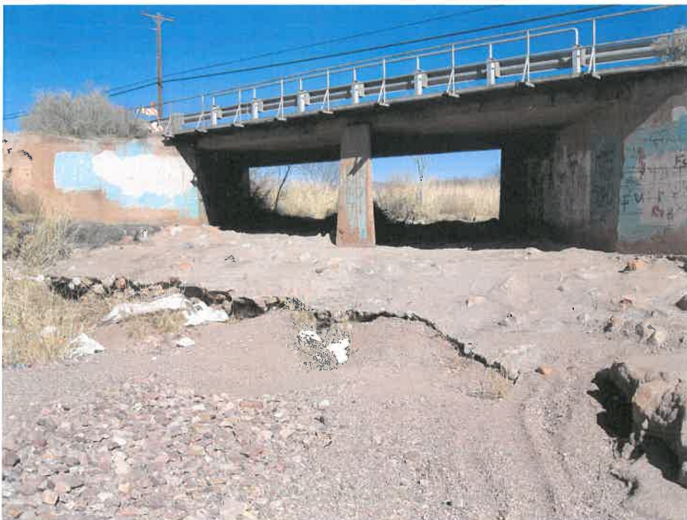
The bridge on N. Sulphur Springs Street.
