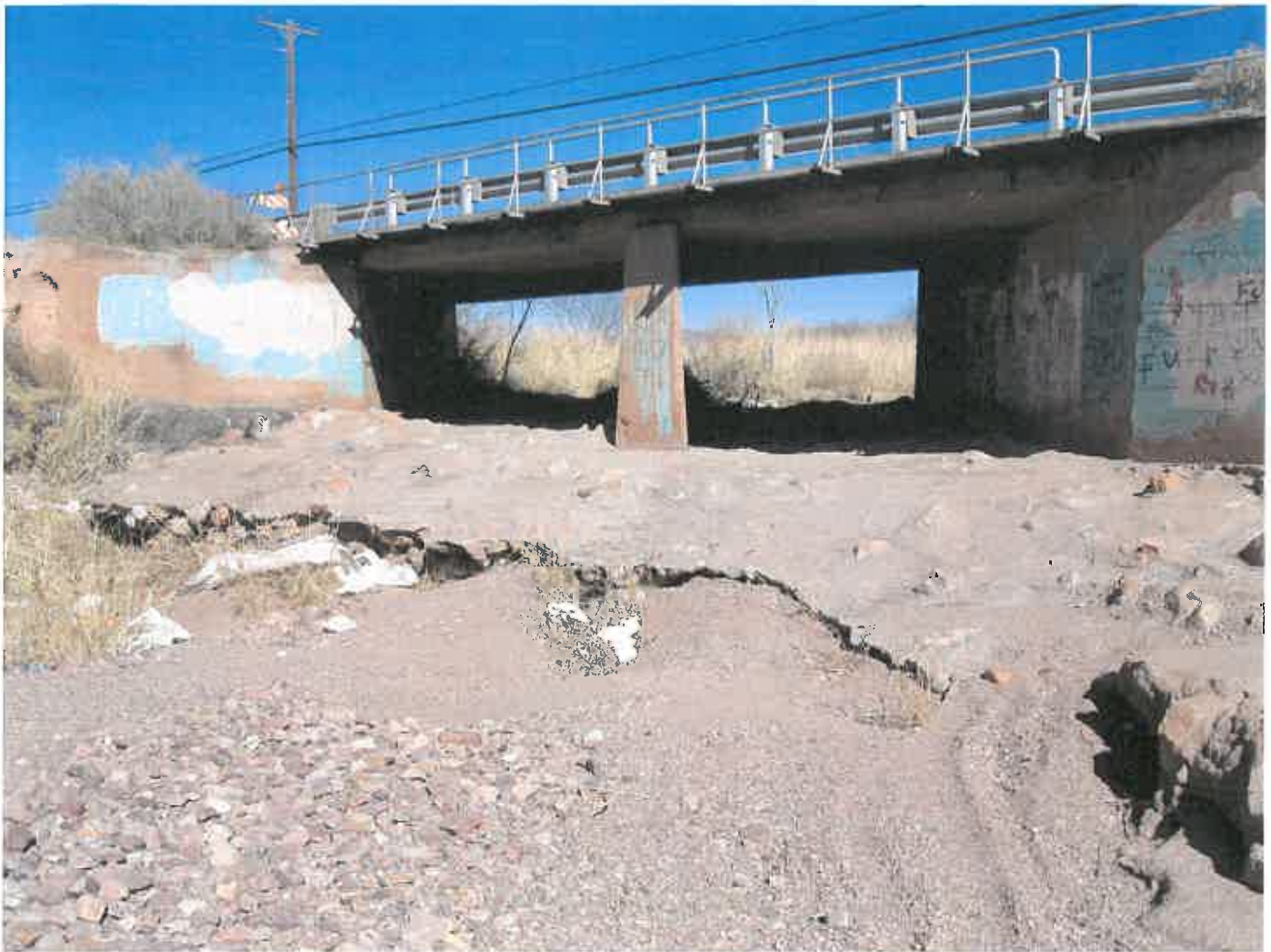
The bridge on N. Sulphur Springs Street.
