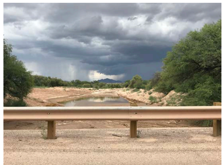
Wash along southern property boundary
