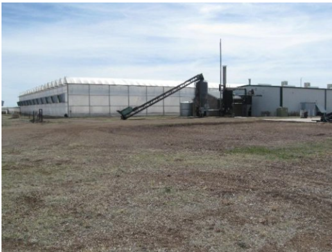
View of greenhouses and shop
