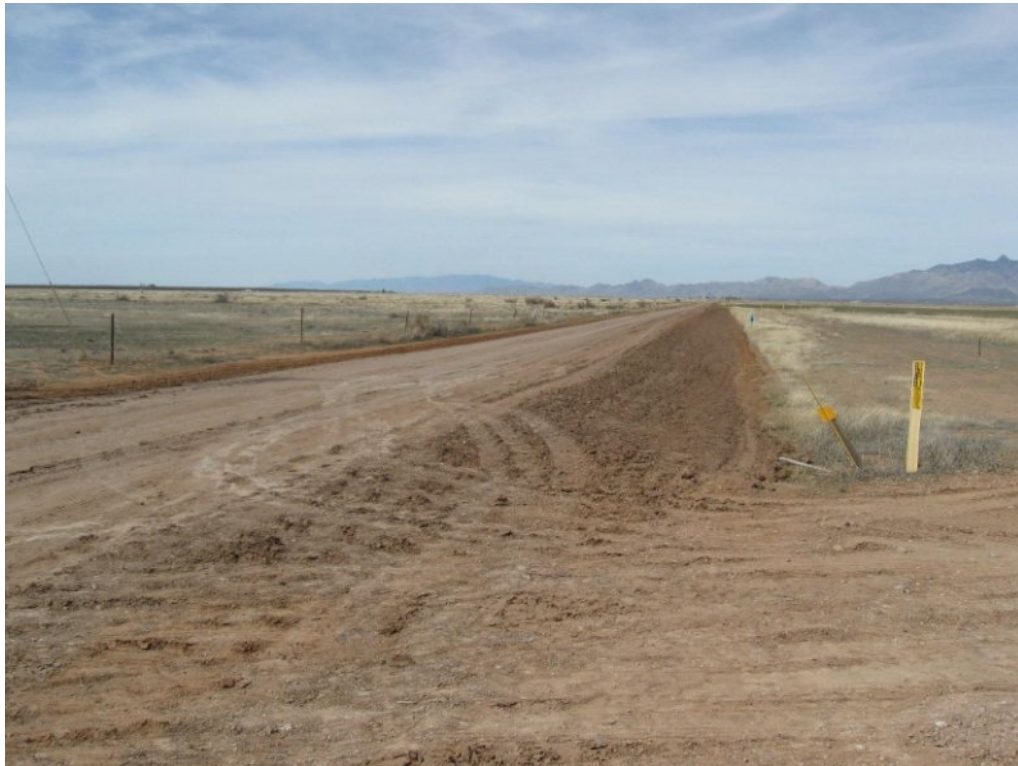
View of prep work on Bell Ranch Road
