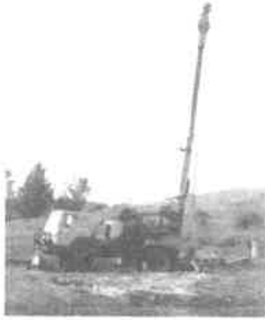
Modern truck-mounted drill rig
