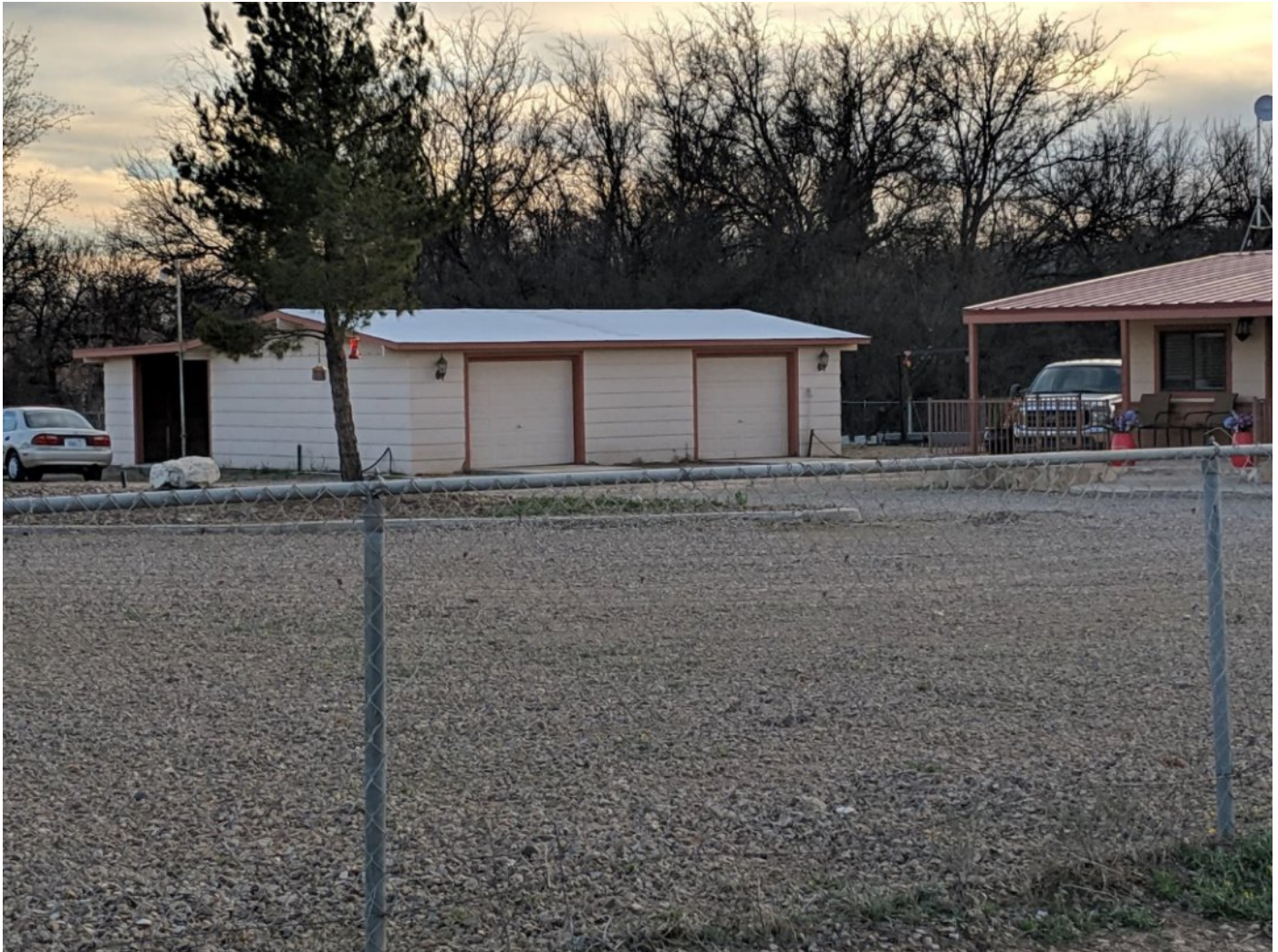
Existing garage, new garage located to the right, behind the home
