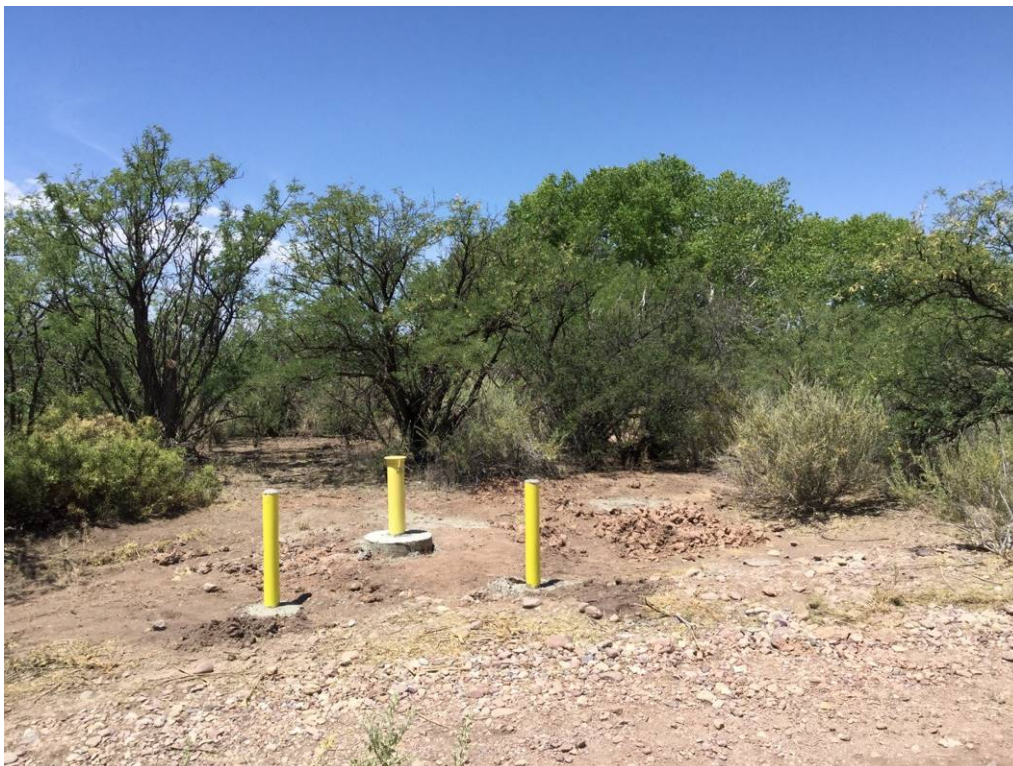
PHOTO 20: LOOKING WEST, DIRECTLY AT MONITORING WELL. (PHOTO POINT 7)
