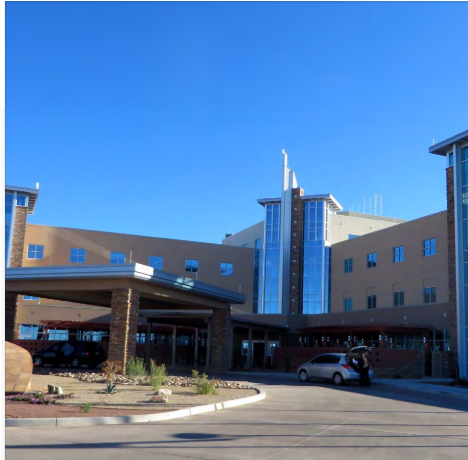
Canyon Vista Medical Center
