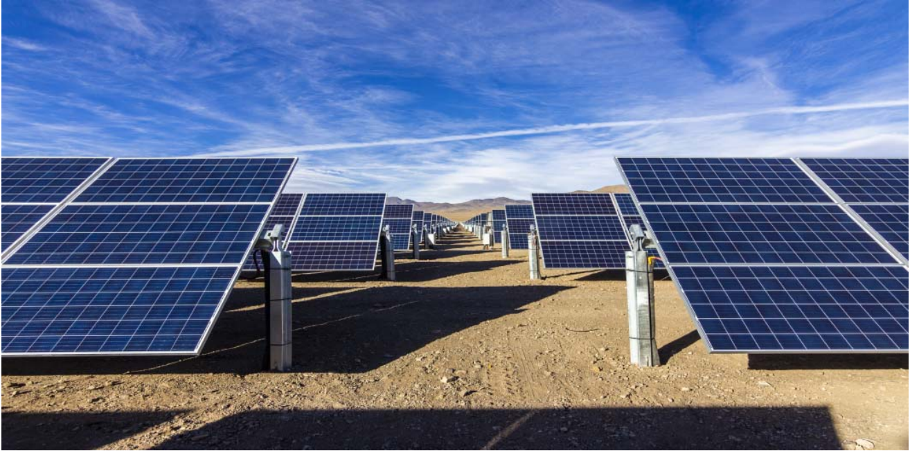
Figure 7: Typical ground mounted solar field
