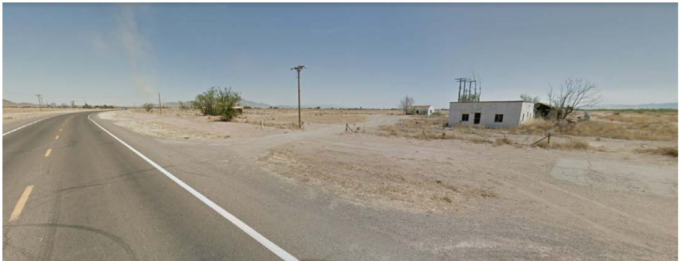
Figure 4: Site Photo 1 (Looking southeast from Ft. Grant Road, vacant and dilapidated structures shown)
