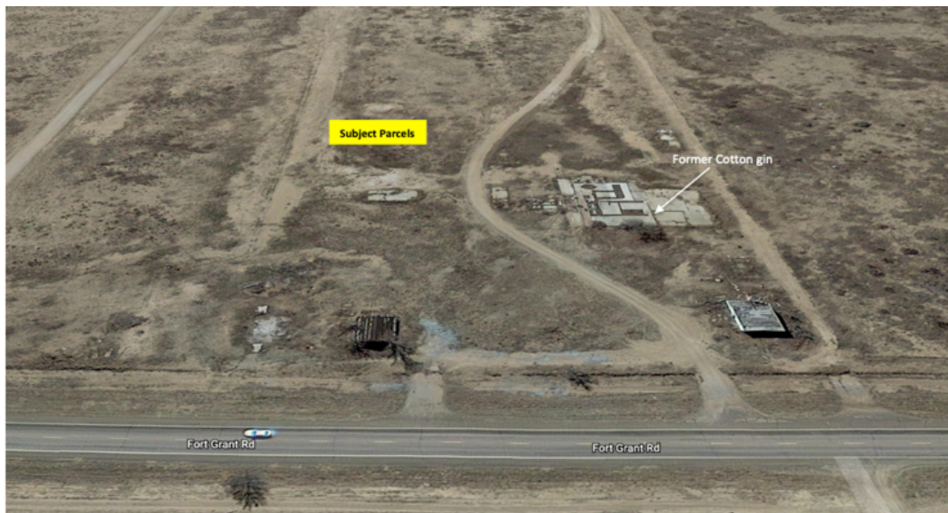
Figure 4. View of the Parcels and proposed site access point from N. Fort Grant Rd. (POV: looking South)
