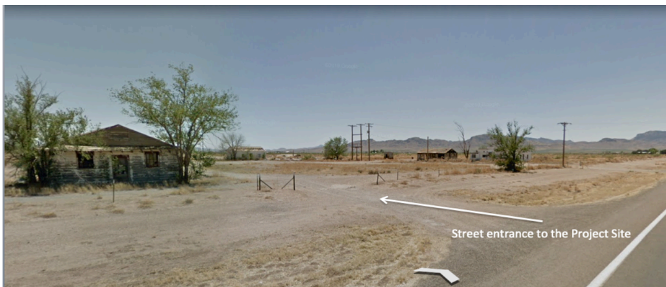
Figure 3. View of dilapidated cotton gin buildings from N. Fort Grant Rd (POV: looking to SW)
