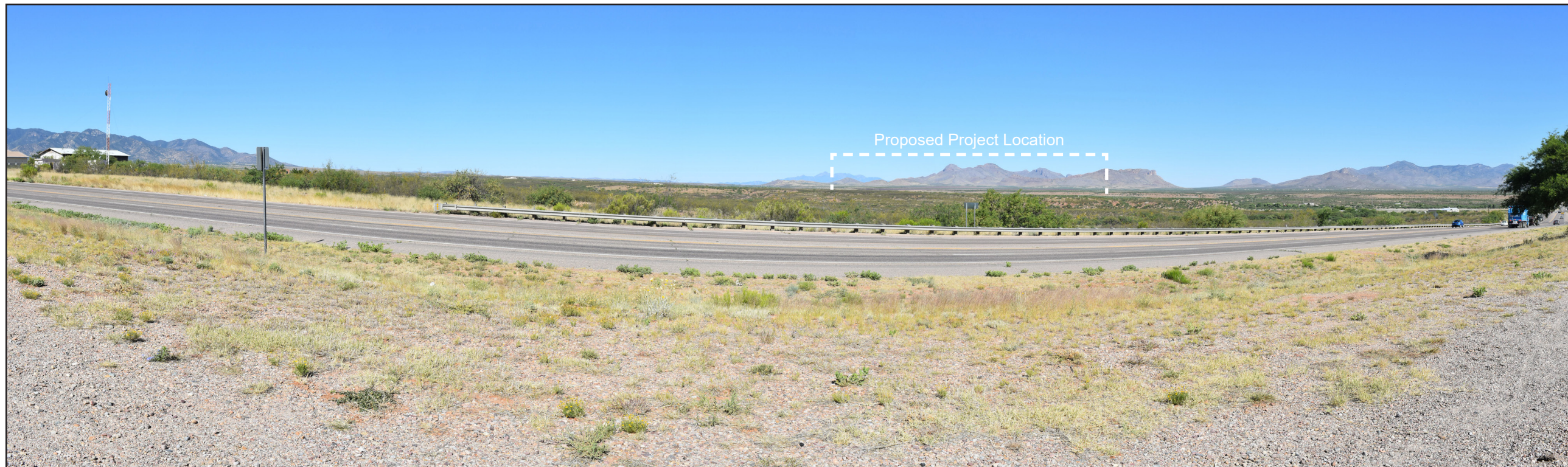
KOP 4 - Proposed Project: Huachuca City municipal buildings, looking west
