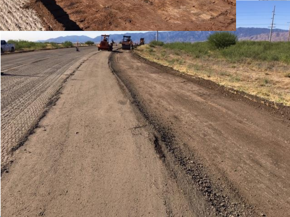
Subgrade fix north end of project. Remove additional 12" subgrade and replace with millings.
