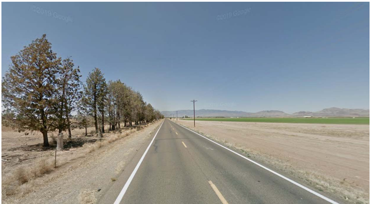
Figure 6: Facing north on Ft Grant Road from the intersection of Ft Grant Road and W Dry Tumbleweed Lane. The western side of the road has a fairly consistent line of planted shade trees.
