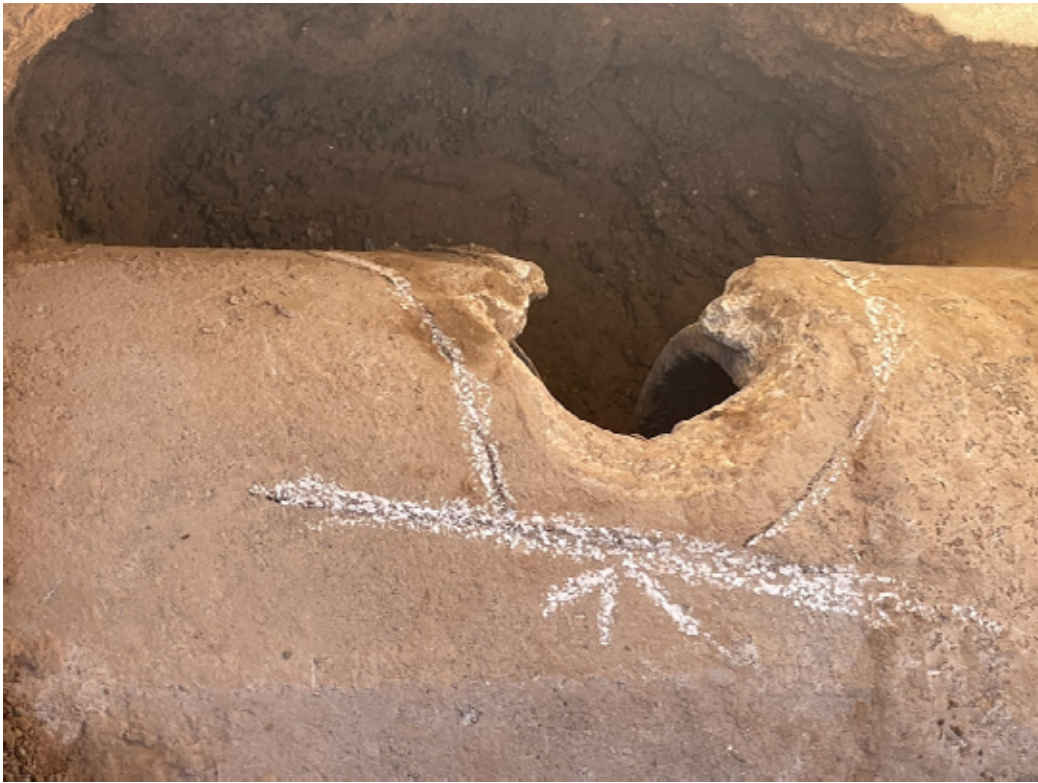
CO1.7 Pipe Repair
