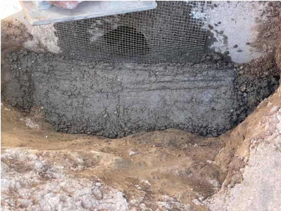
CO1.7 Pipe Repair
