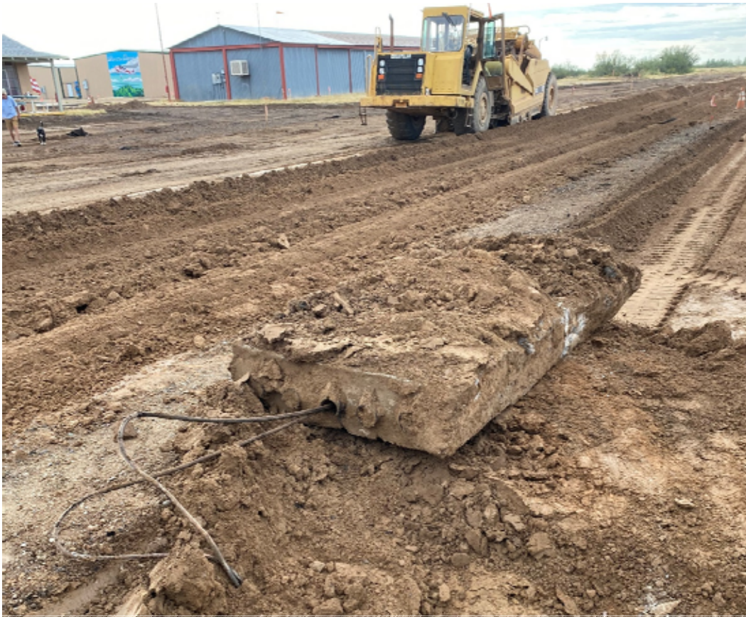
CO1.3 Concrete Encased Duck Bank Removal
