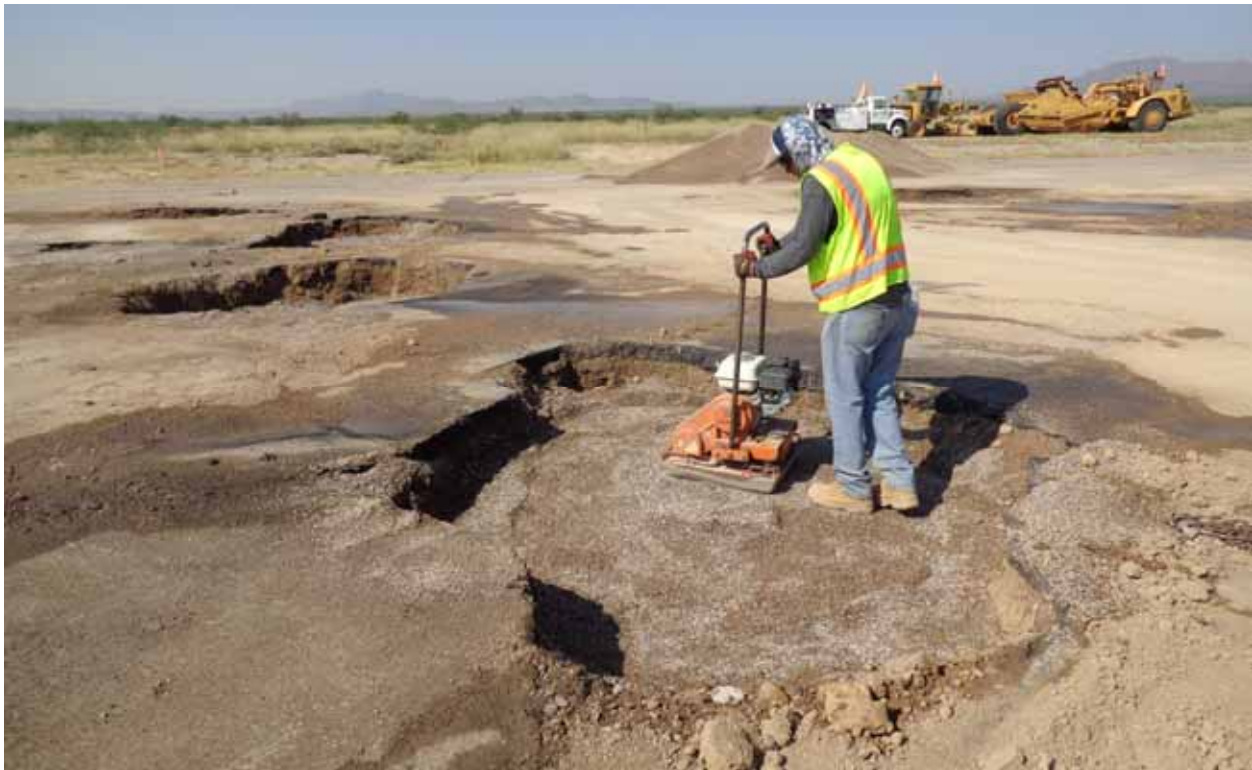
CO1.1 Backfill Placement and Compaction
