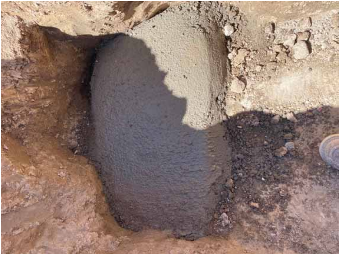
CO1.7 Pipe Repair
