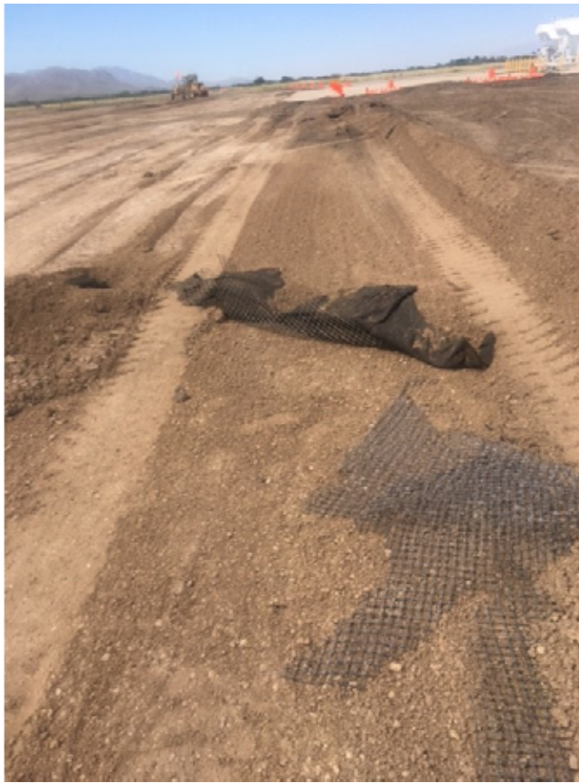
CO1.5 Fabric and Geogrid Found
