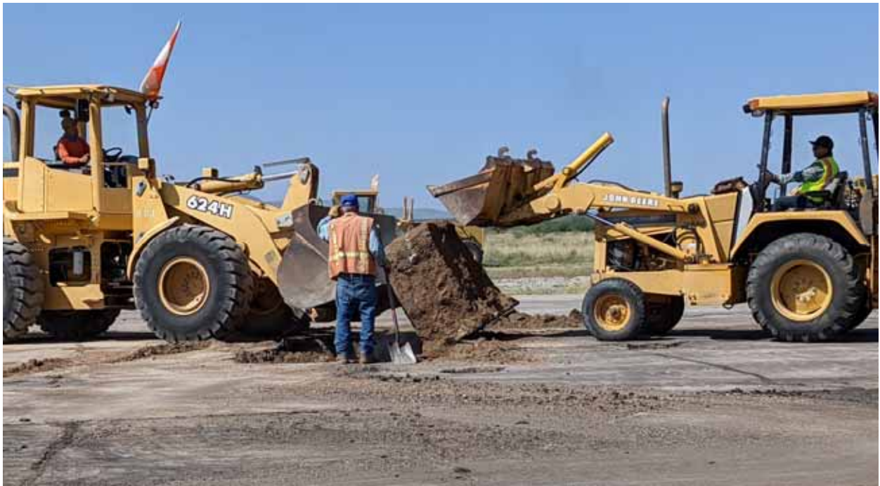
CO1.1 Concrete Block Removal
