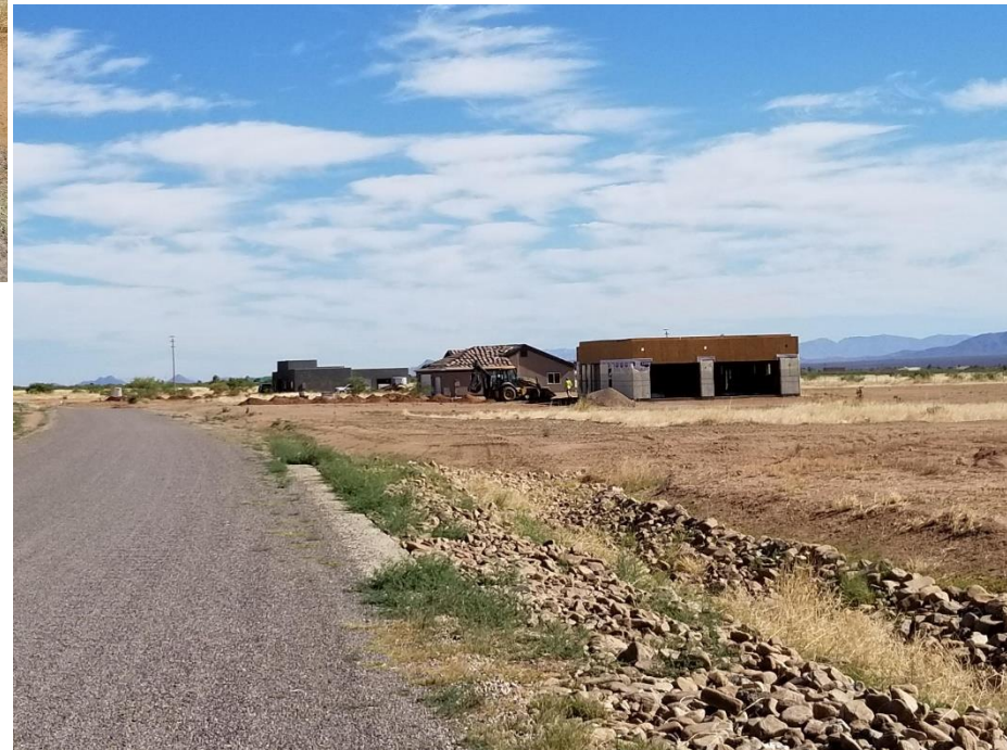
Homes under construction on Caballero Loop
