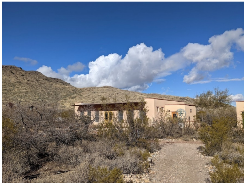
Photo 8: Existing building at Diamond Mountain
