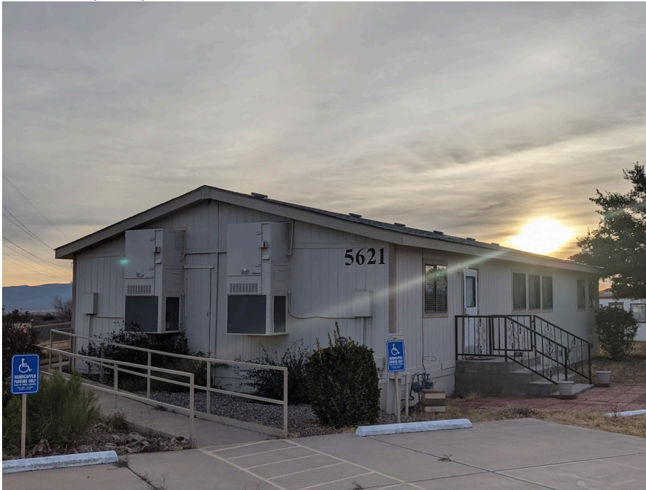
Concrete parking and ADA access
