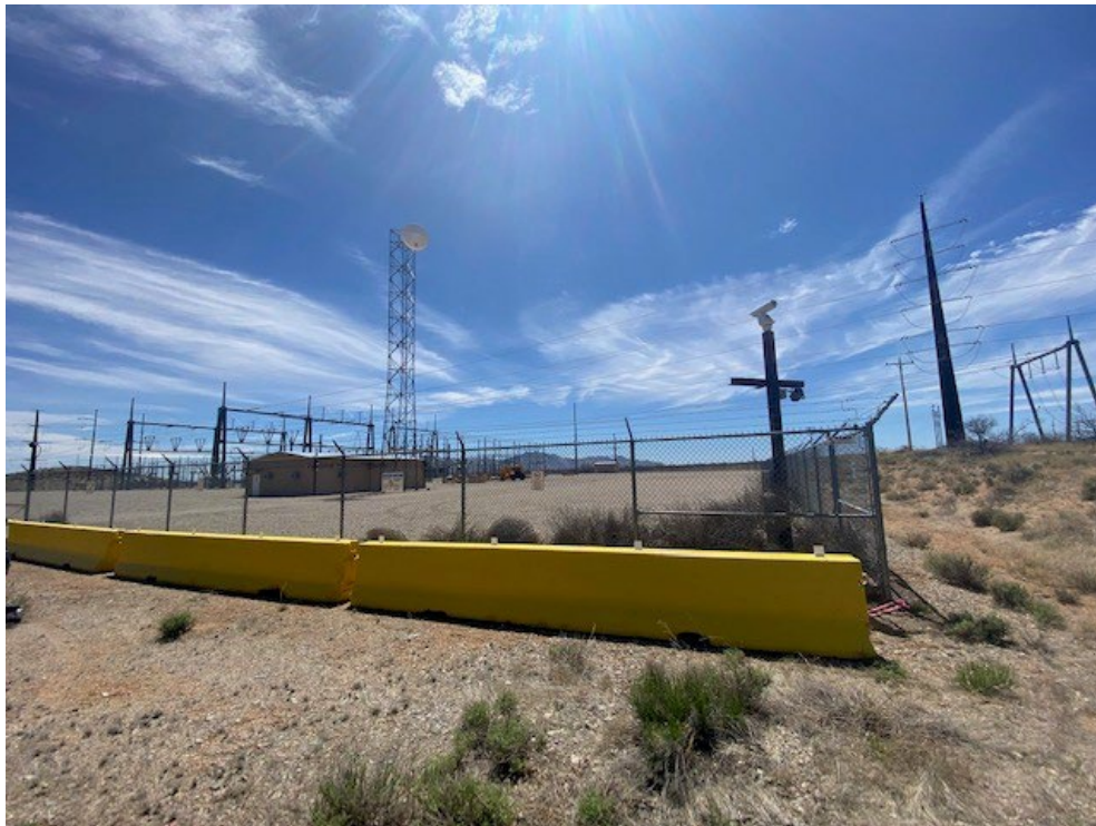
Current facility with chain link fence
