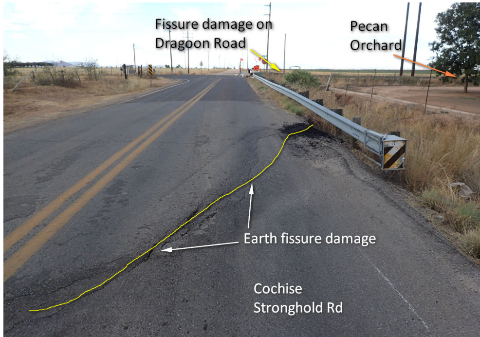
Figure 5.3-14. Earth Fissure Formation Cochise Stronghold Road
