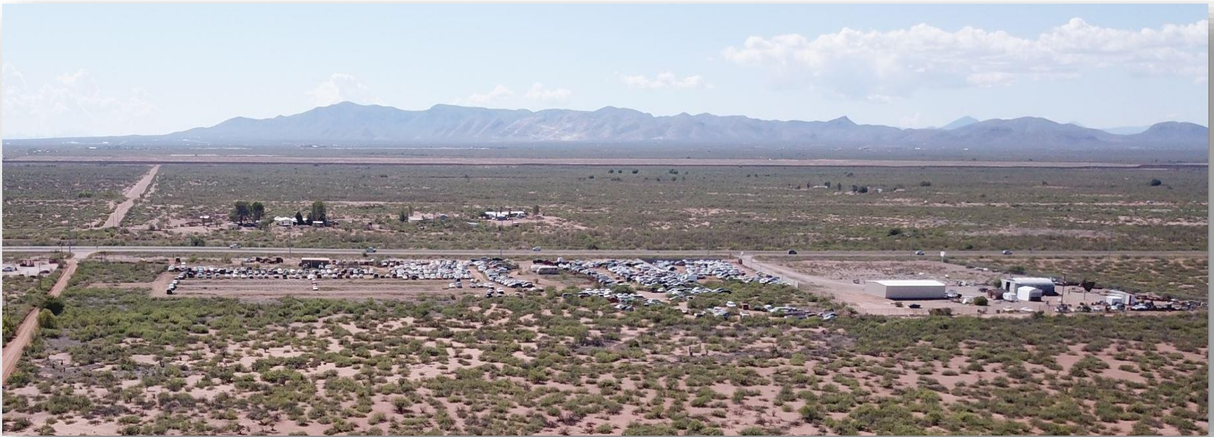
Commercial properties to south
