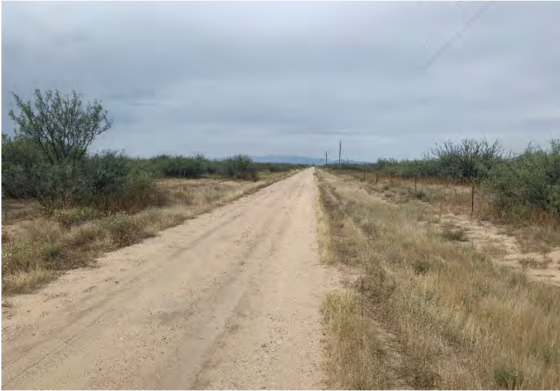
Photo 19. Feature: N/A OHWM: No Width: N/A View: North Notes: Dirt roadway along the eastern boundary of the northeastern portion of the Analysis Area.
