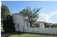
A small false front building.
