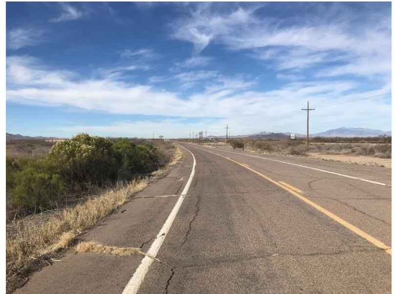
I-10B, viewing west
