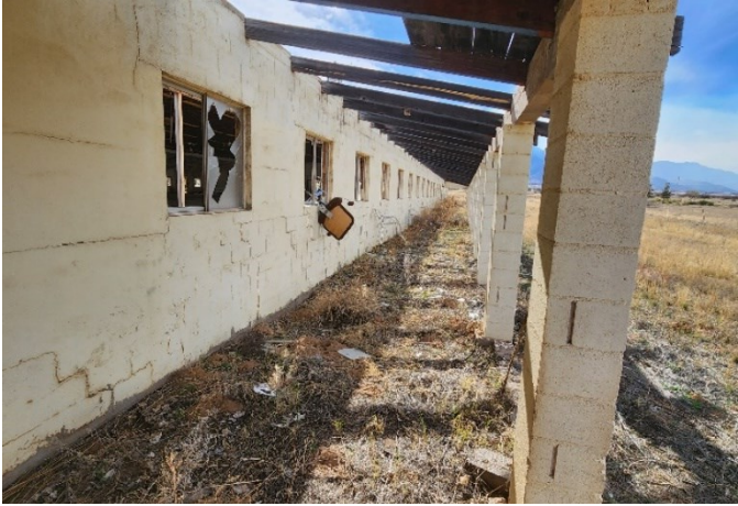
Exterior View Under Overhang
