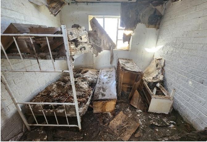
Girls Dormitory Typical Dorm Room View
