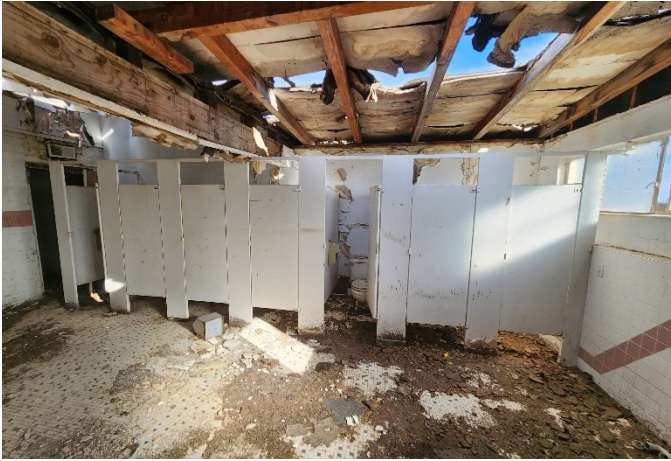
Girls Dormitory Restroom View
