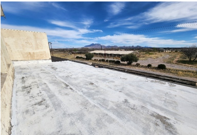
Flat Roofing Around Dome
