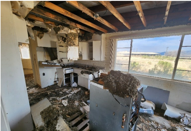
Girls Dormitory Kitchenette View
