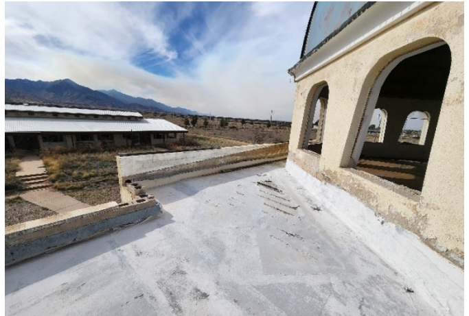
Overall Roof Deck View Around Dome
