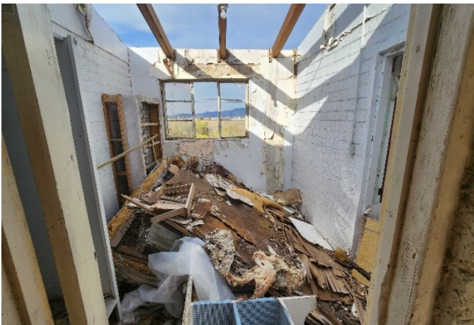
Boys Dormitory Typical Dorm Room View
