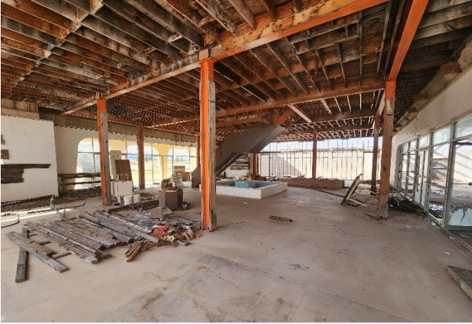
Overall Interior Lobby View
