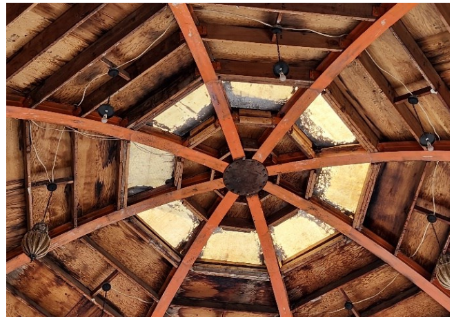
Interior View of Dome Compression Ring
