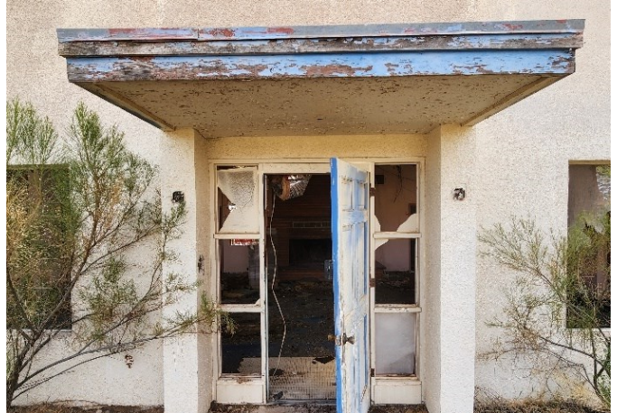
Girls Dormitory View of Front Entrance
