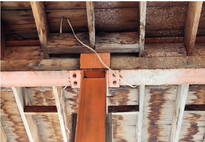
Steel Column Attachment at I-Beam
