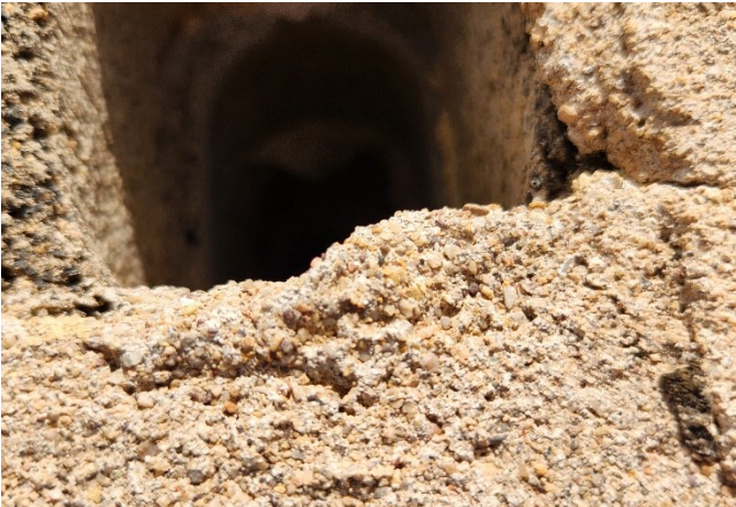
Closeup Non-Reinforced Masonry
