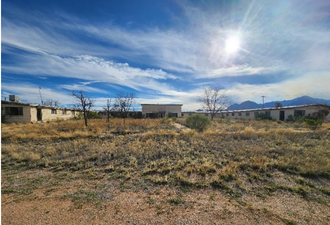
Overall Girls Dormitory Exterior Front View
