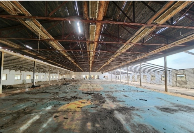
Overall Interior View of Main Auditorium
