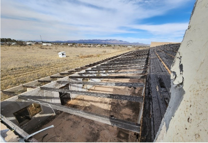
Exposed Rafters on North Wing
