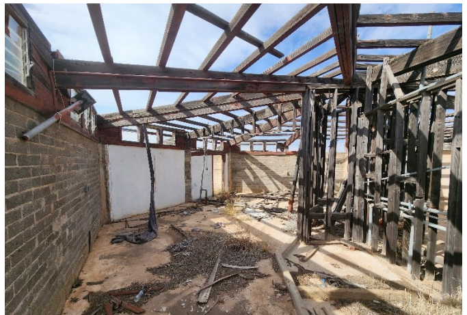
Overall Interior View
