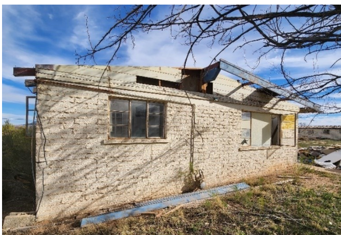
Overall Boys Dormitory Exterior View
