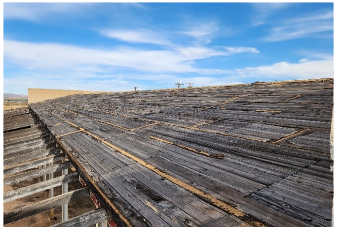
Exposed Roof Decking
