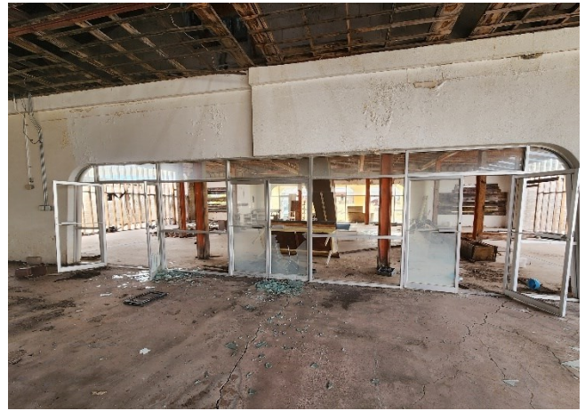
Main Entrance Glass Panels and Doors
