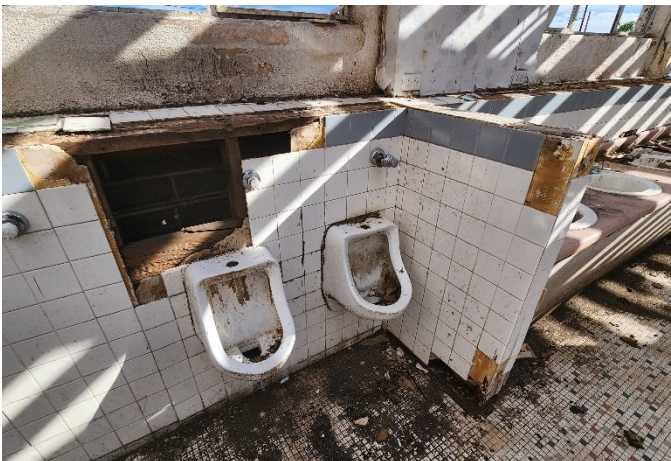
Boys Dormitory Restroom View
