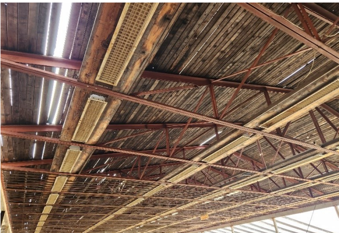
Overall View of Steel Roof Trusses
