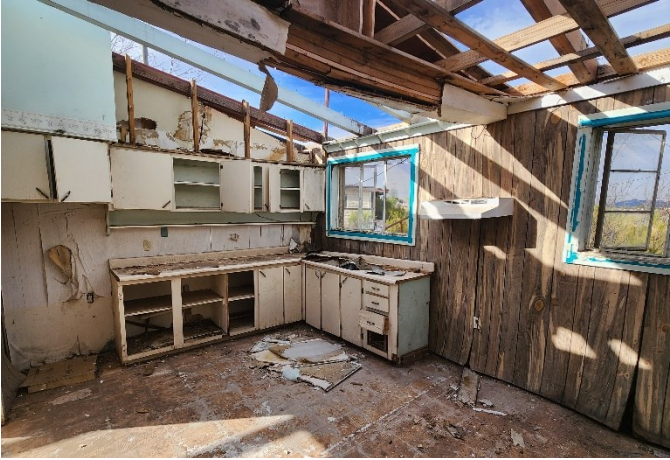
Boys Dormitory Kitchenette View
