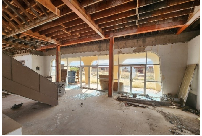
Overall Interior Lobby View
