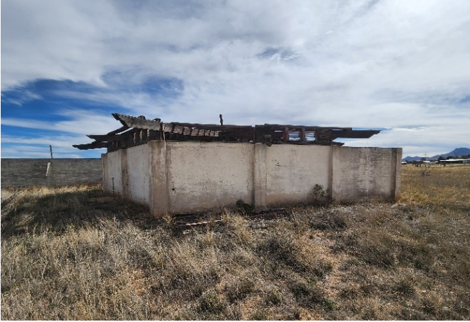
Overall Exterior View
