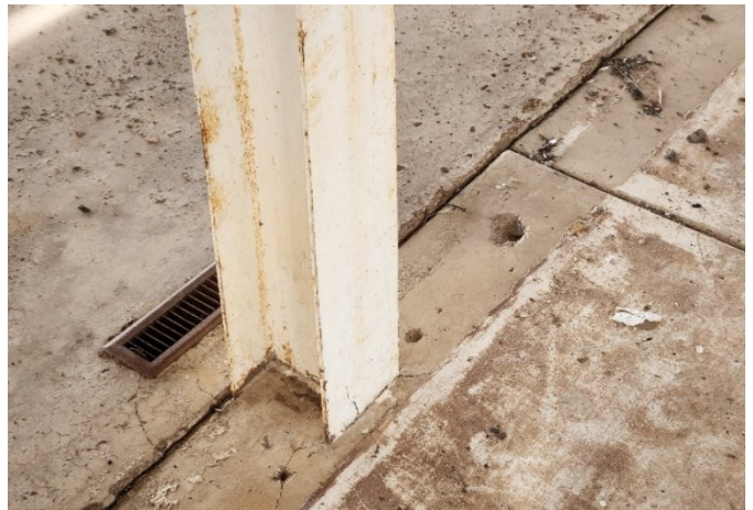
Steel Column Attachment to Floor
