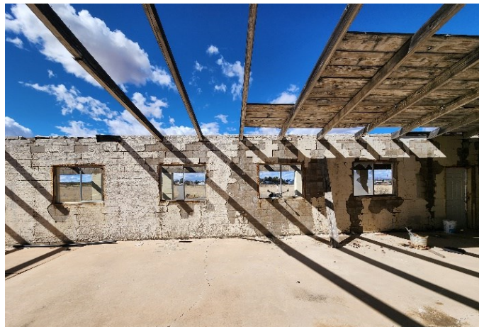
Overall Interior View of Open Roof
