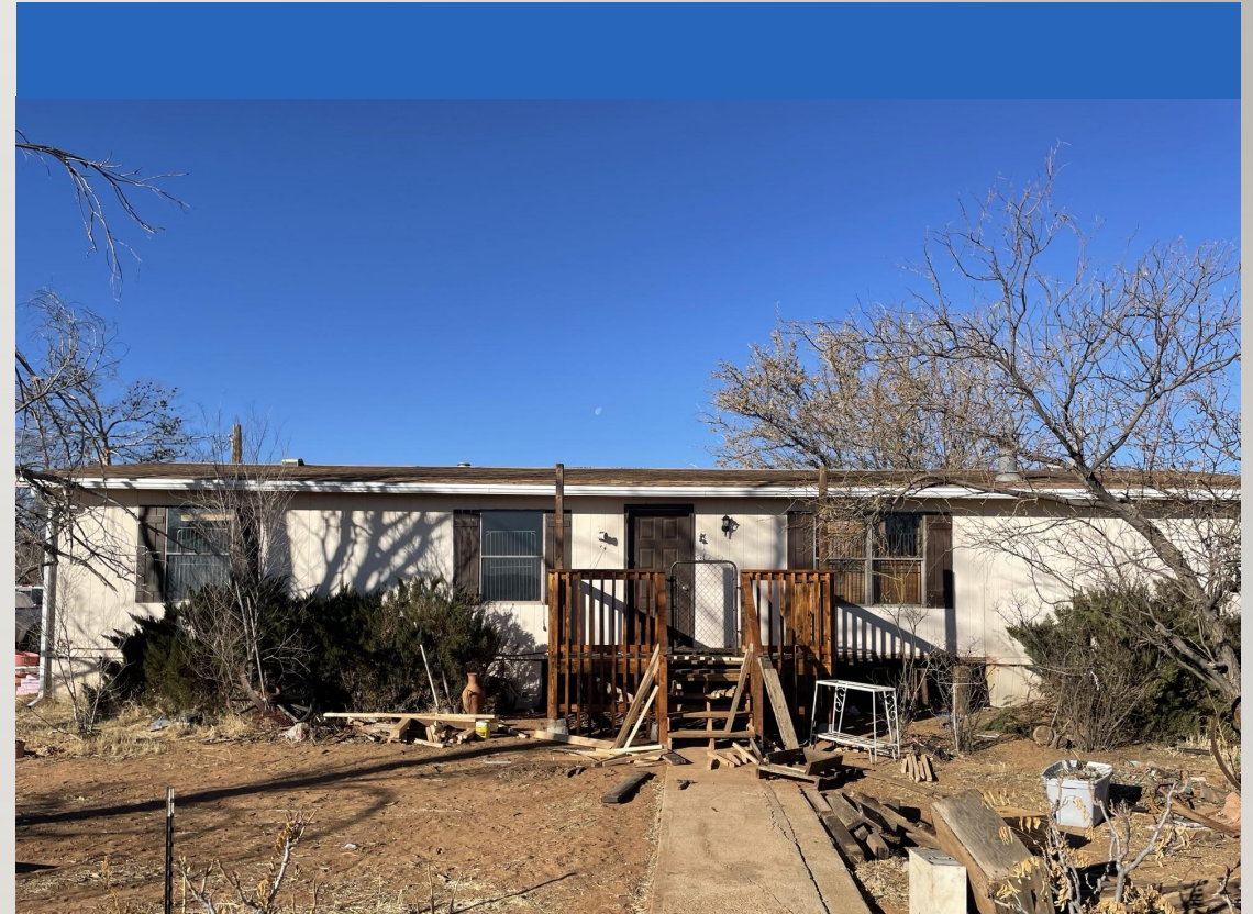
Roof and Deck Replacement
