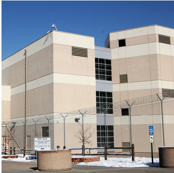
Adams County Detention Facility Replacement, Brighton, CO.
