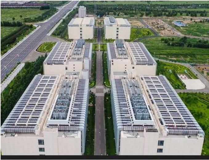
Lakeside Technology Center (Chicago, IL) is a 100 MW facility covering 25 acres.
