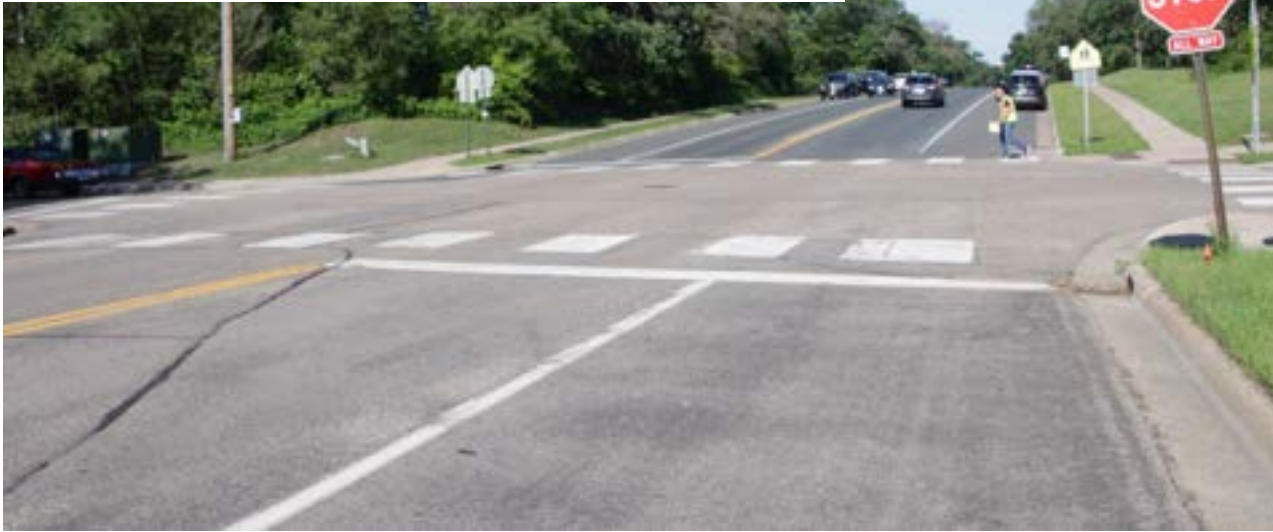
Before Project: 121st Ave. NW & Olive St.
