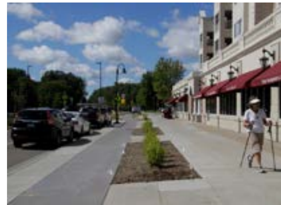
▲ Curb separated cycle track with landscaped buffer space between the protected bike lane and sidewalk. (Richfield, MN)
