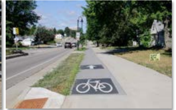
▲ Curb separated directional (one way) cycle track adjacent to sidewalk. (Richfield, MN) When placed adjacent to the sidewalk, a detectable surface should be placed at the edge of the bike lane for people with vision impairment.
