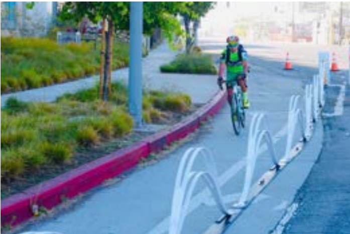
Lower-Cost Protected Bike Lane (also called separated bikeway)
