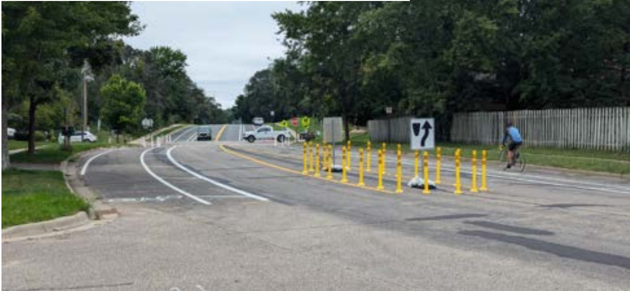
After Install: 121st Ave. NW & Norway St.
