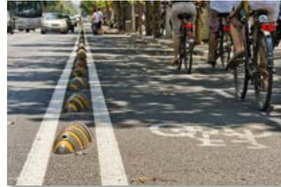
▲ Temporary two-way protected bike lane using a painted buffer space and armadillos to create vertical separation.
