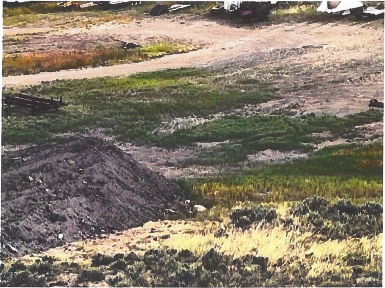
Push pile of dirt cut out from the hill on the SE corner. Note the green stake and manhole cover at the edge of this pile. It appears this dirt is right on top of the sewer line that cuts across this corner. No engineering and geological study was done on the impact of grading into this steep hillside. Looking down slope from 913 Ridge Dr.
