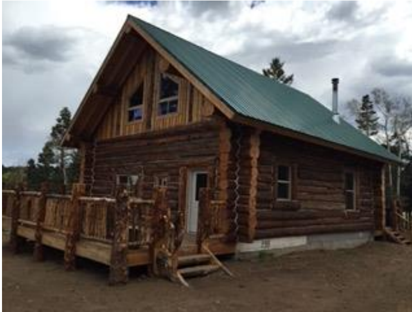
Photo 1 Swedish Cope Log Home by Independent Log Company
