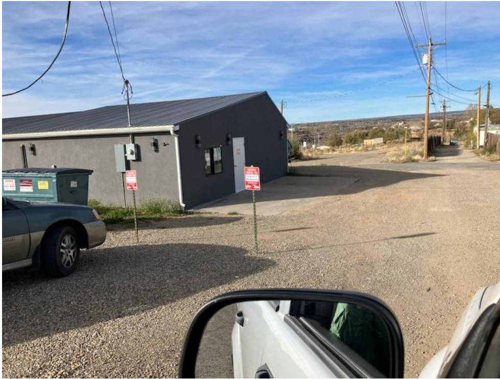
Approach to drive-up window from alley heading north
