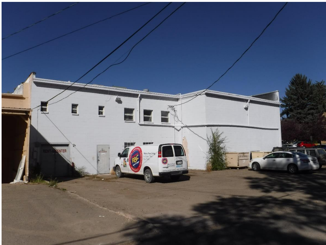
5MT22591 Rear Façade Oblique View Looking Northeast
