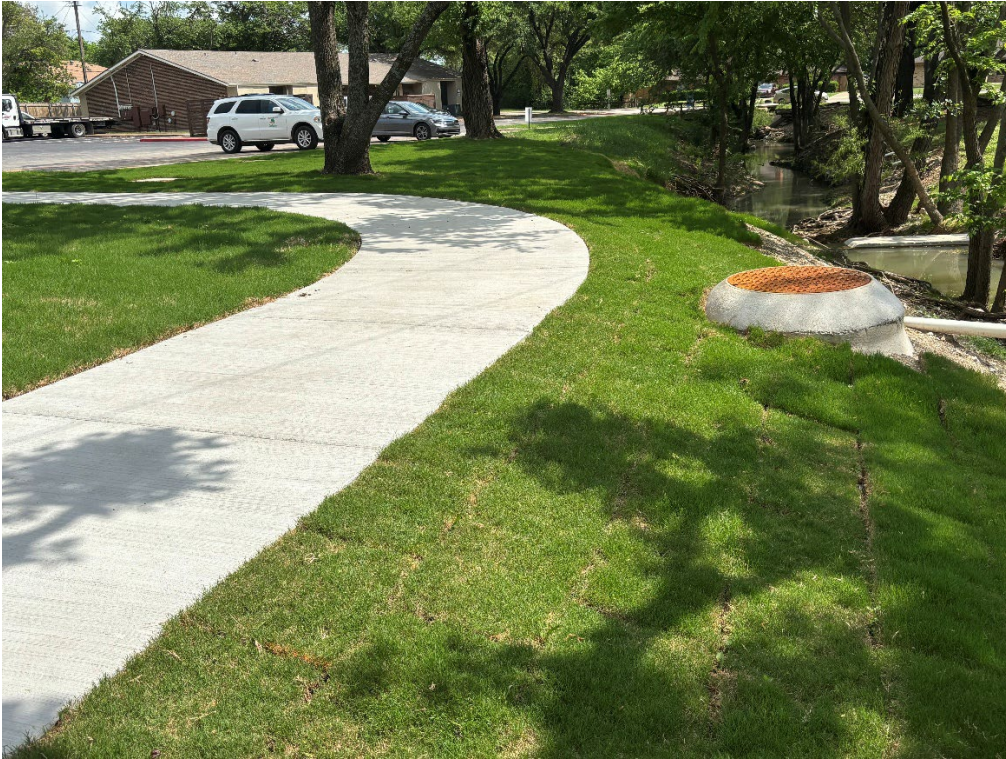
Fig. A6. Sidewalk and Sodding installed
