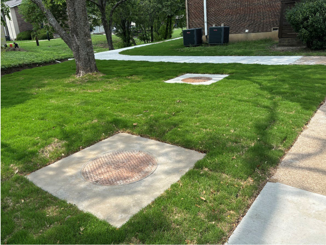
Fig. A4. Standard 5-foot Manhole installed.
