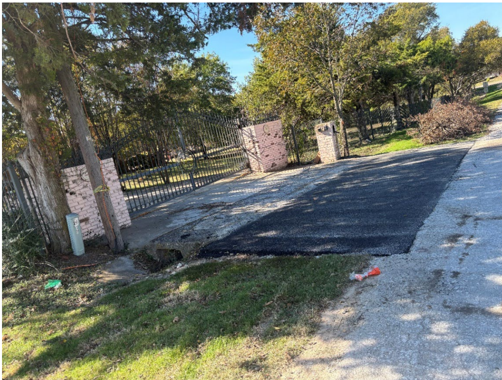
Fig. A2. The Asphalt Driveway restored after sewer line installation
