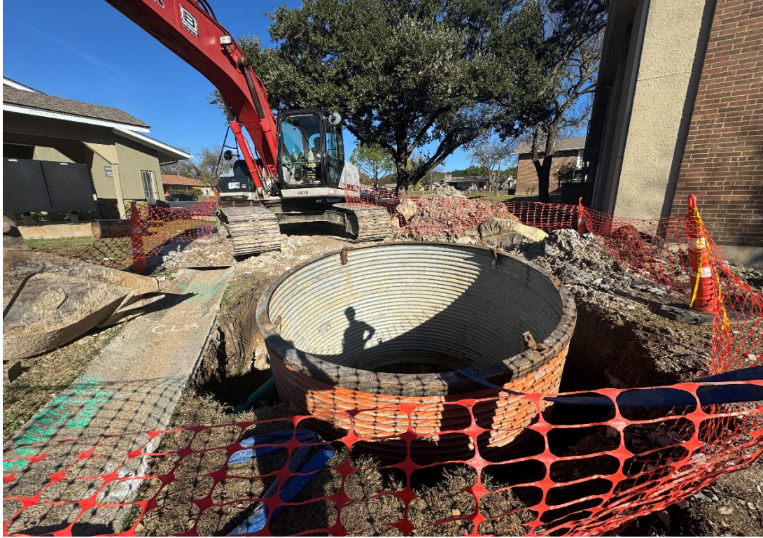
Fig. D1. Sanitary Sewer Manhole Installation Within Riverbend Apartments in progress
