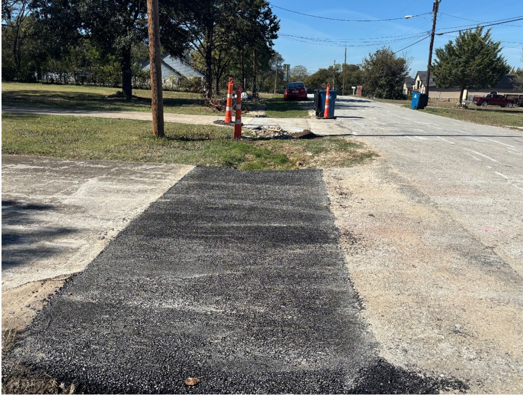
Fig. A1. The Asphalt Driveway restored after sewer line installation
