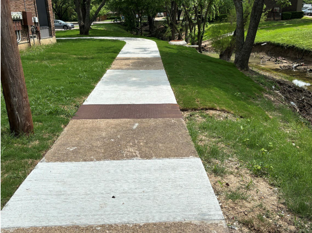
Fig. A7. Sidewalk and Sodding installed
