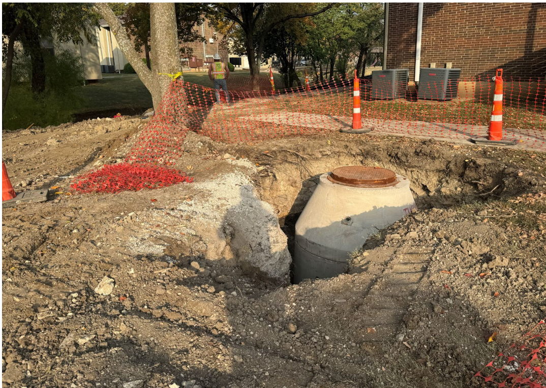
Fig. D2. Sanitary Sewer Manhole Installed Within Riverbend Apartments in progress
