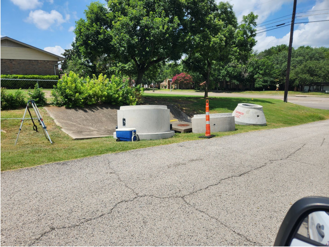
Fig. B1. Before construction photo
