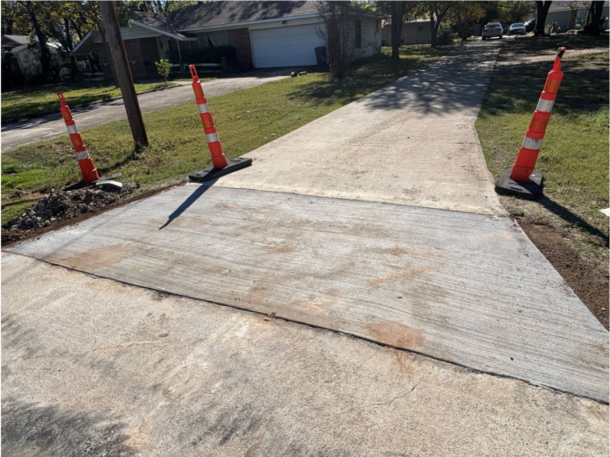
Fig. A3. The concrete Driveway restored after sewer line installation
