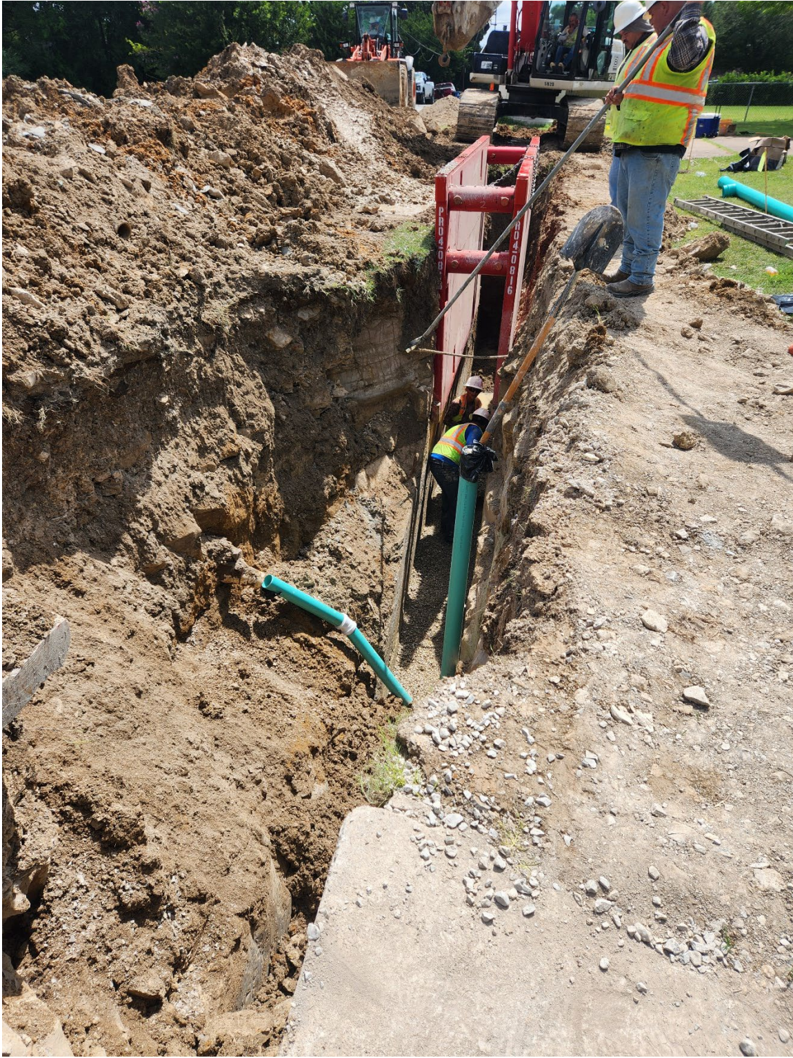
Fig. D3. 8 - inch sewer line installation along Reedsport Place in progress
