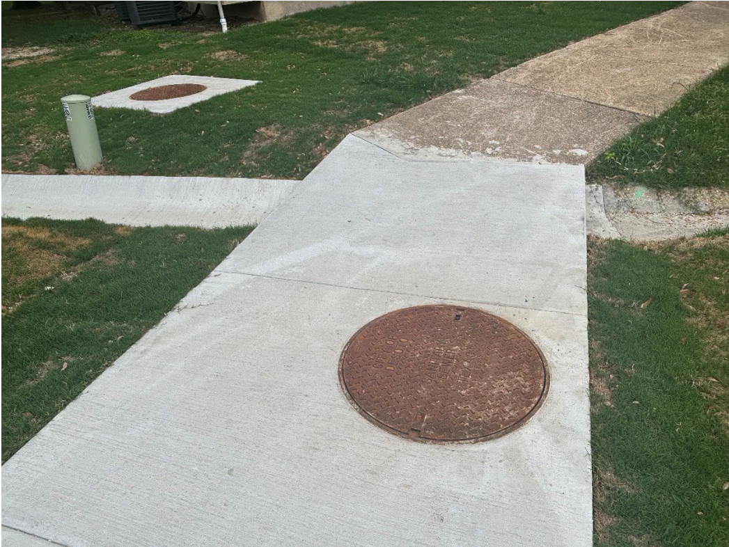
Fig. A5. The Standard 5-foot Manhole installed and the flume restored
