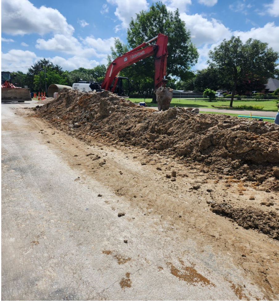
Fig. D4. 8 – inch sewer line installation along Reedsport Place in progress
