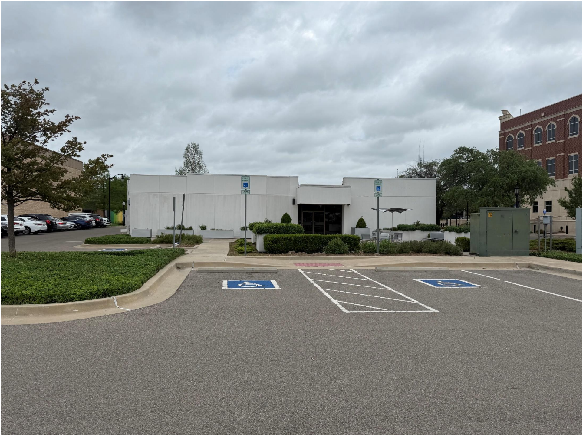
Location - south wall of 24 E First Street
