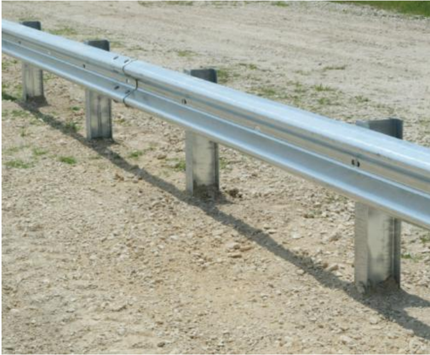
metal beam guardrail
