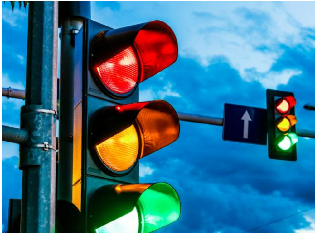
traffic signal system
