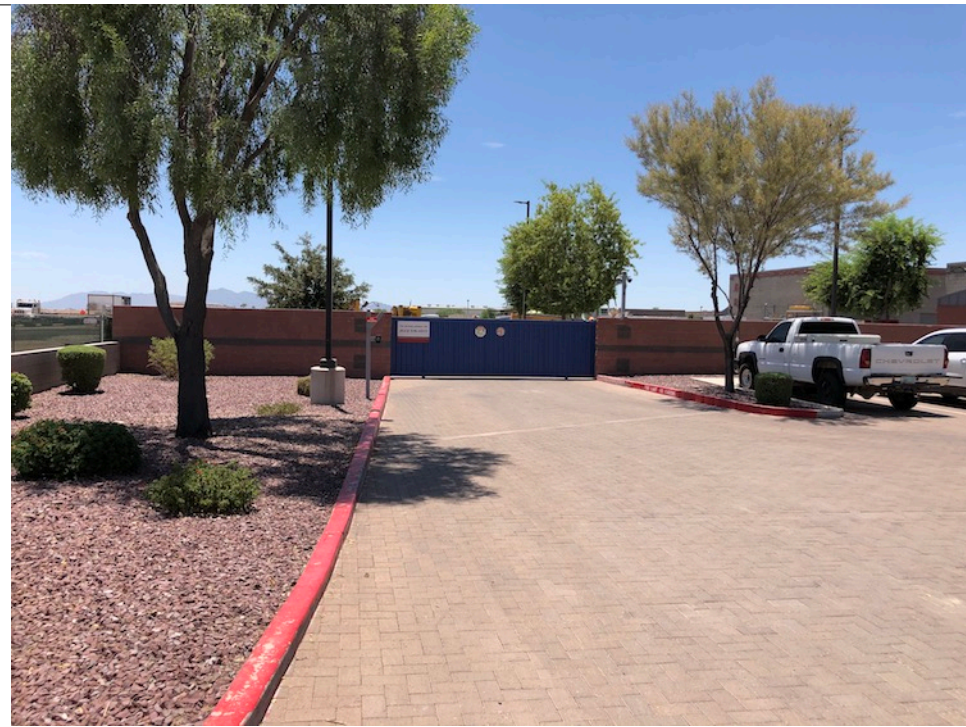
PHOTO 1: EXISTING SOUTHWEST CONCRETE GATE AND MASONRY WALL THIS PROJECT TO COPY COLOR SCHEME AND MATERIALS
