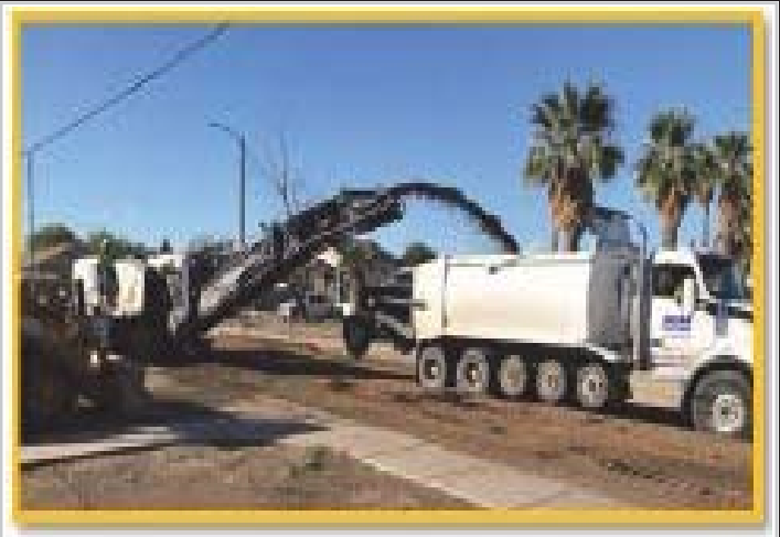
"A" Street Project
