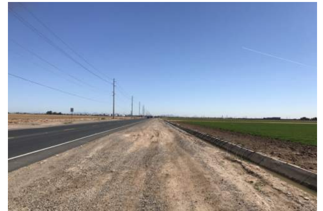
View to the east along West Olive Avenue from the NEC of the subject property.
