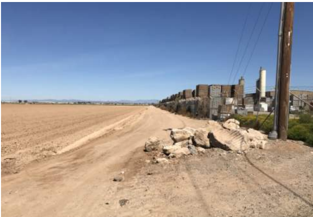
View to the north along the eastern site boundary, from near the SEC of the subject property.
