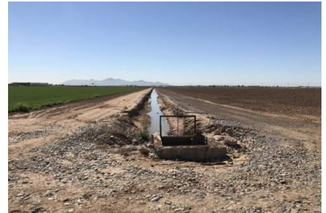
View to the south along the irrigation canal running north to south in the middle of the subject property.
