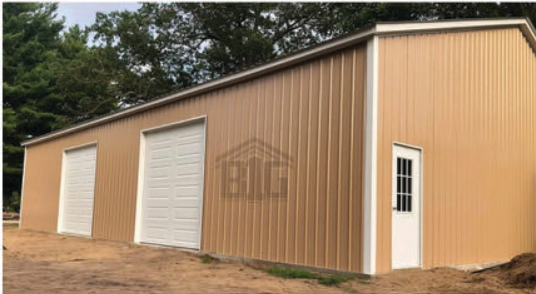
Photograph of actual building similar in size and style
