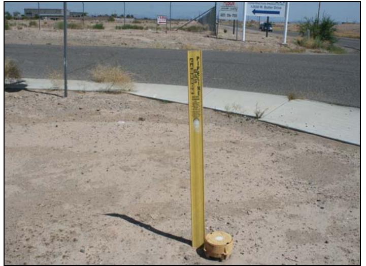
This view shows the Southwest gas line utility marker on the northeast corner of the site.
