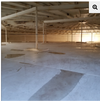
Canterbury Water Tank
