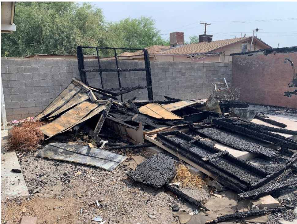
Large Shed that has been destroyed by fire damage.
