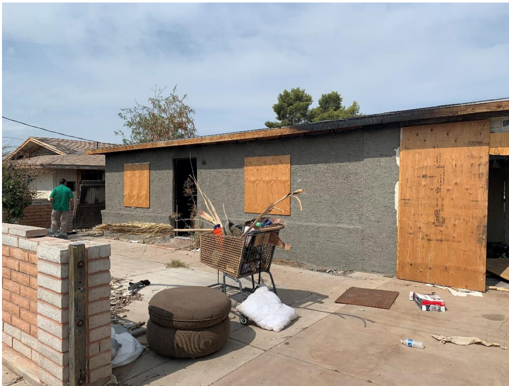
Front view of main structure. Front door unsecured.
