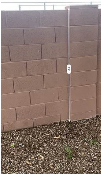
Height of the current wall want to rise to approx. 8ft
