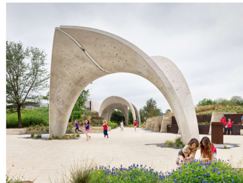
Rainwater Harvest Archway
