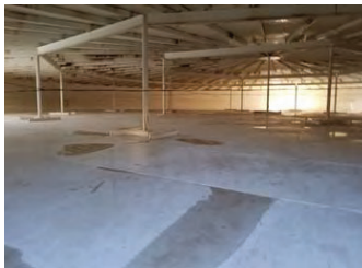
Canterbury Water Tank
