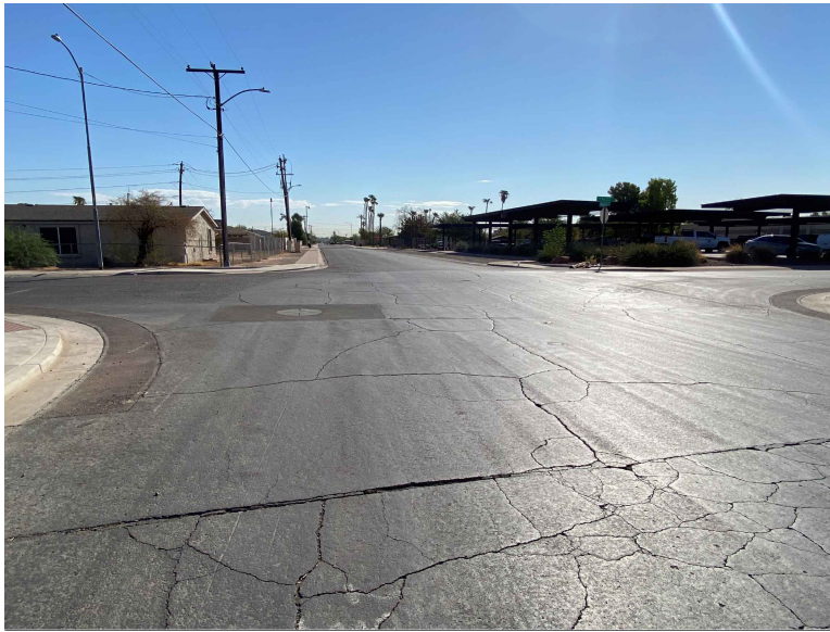
Photo 4 - Ventura Street at 1st Avenue (Looking East)
